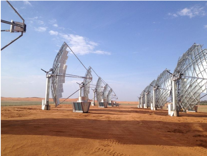
Construction progress as of January 2014
